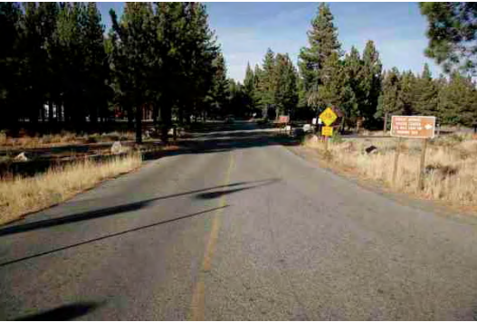
Photo #2 Notes Condition photo
