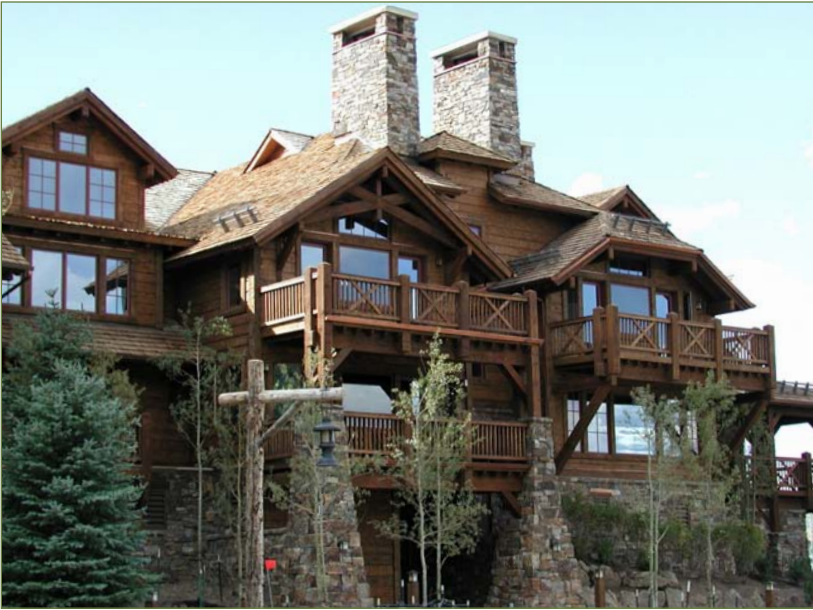
Figure 3.3: Detailing at railings and structural components reflect
