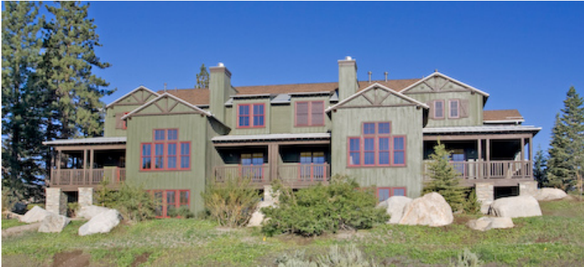
Figure 3.7: Roofs utilize simple gable forms
