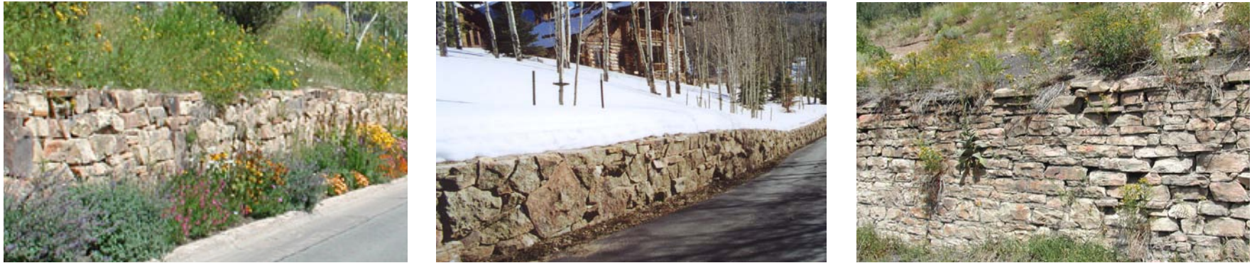
Figure 2.2: Retaining wall designs should have a dry-stack appearance
