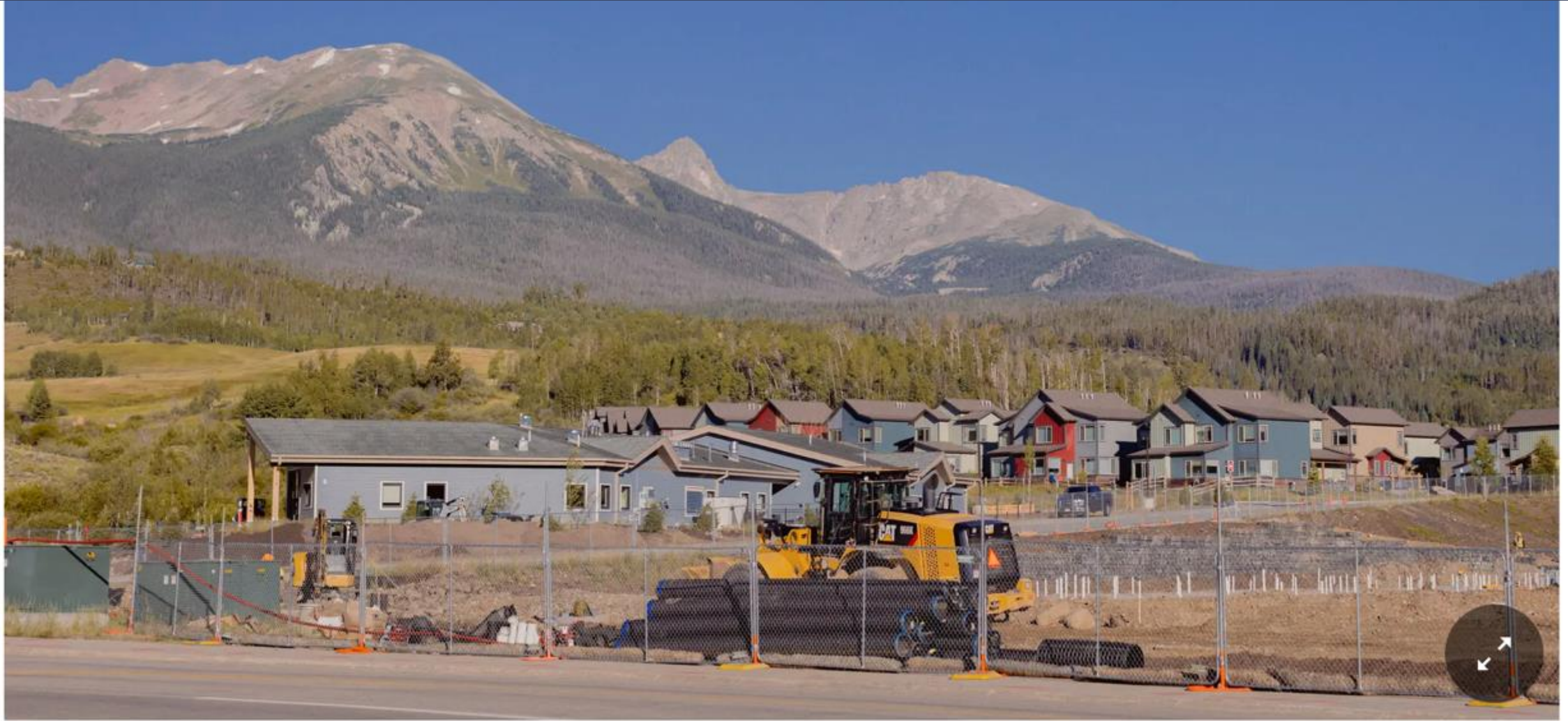
A construction site in Silverthorne, Colo. Some officials and residents in the area have acceded to limited construction but are wary of adding taller, dense multifamily buildings.
