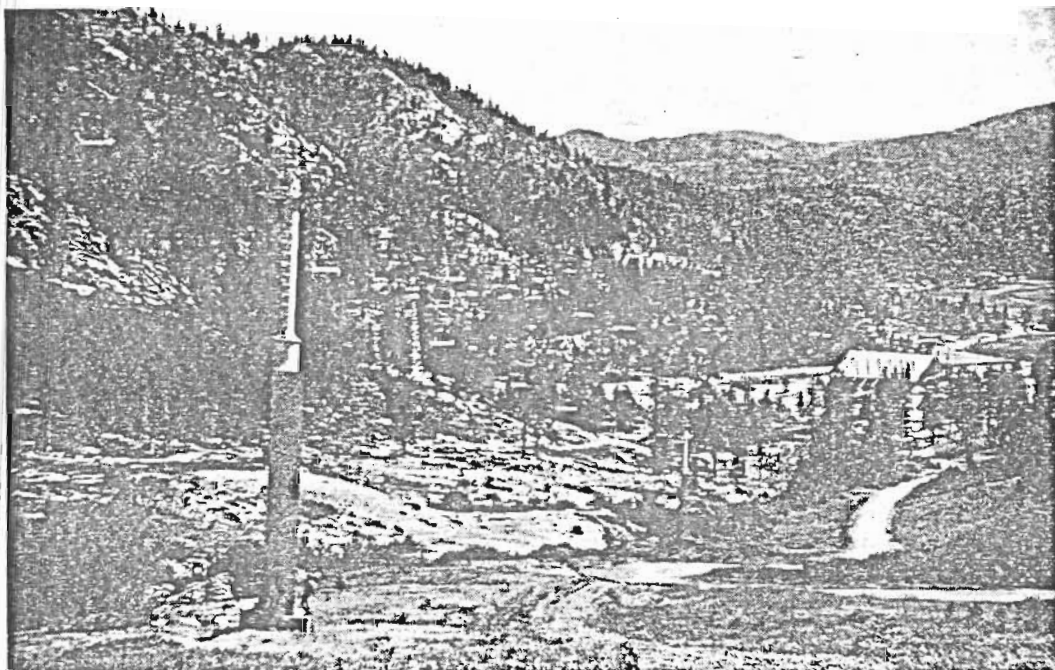
Figure 7. This lift passes above an avalanche runout zone. Note that the very tall towers at the ends of the span are protected with steel vees due to their locations at the edges of this large avalanche. Person at bottom of tower, on left, gives scale.
