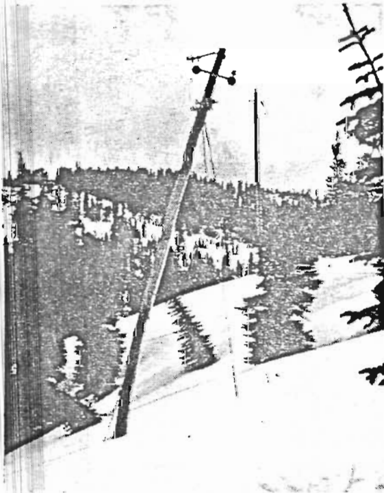
Figure 23. A striking example of snow creep. Creep forces, acting on guy wires on the uphill side of the pole, threaten to break the pole.
