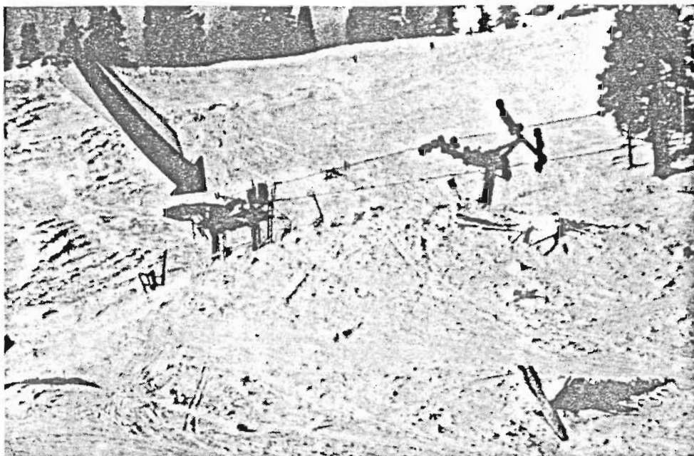
Figure 14. A lift terminal placed in the extreme runout zone of a major avalanche path. Although evidence showed the avalanche had travelled this far sometime in the past, it had not been observed to do this since the area was developed (14 years earlier). Thus, the developer accepted the risk of using this otherwise desirable location.
