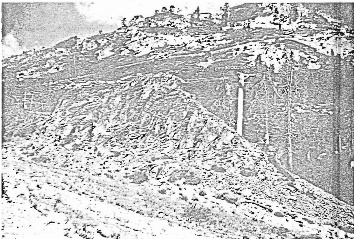
Figure 6. This tower location takes advantage of a large volcanic outcrop for protection from an avalanche to the left.
