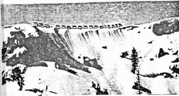
The picture shows an experimental installation featuring several different types of roofs. The last four roofs on the right were not effective.
