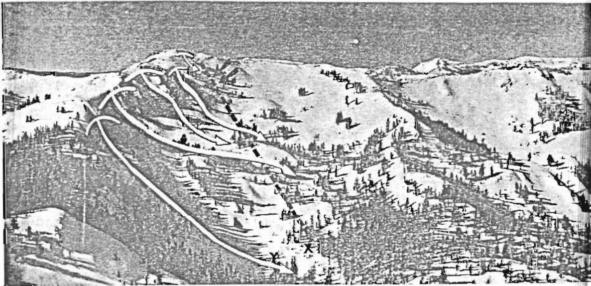
Figure 19. This lift was installed by a ski area that desired a high elevation lift to enhance early season potential. Avalanches from the left forced the ski area to build in a less than ideal lower terminal location (X), as the ideal location (Y) is regularly overrun by large avalanches. High spans were designed into the lift to bridge over avalanches farther up the lift line. Line towers were installed on protected knolls and outcrops. Snow creep is a severe problem at two line towers (black arrows). The upper terminal, although within 200' of the ridge, suffers damage from snow creep and occasional climax avalanches. Thus the planning was not an unqualified success.
