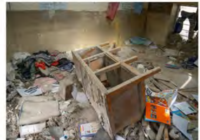
Debris in what's left of Thame's elementary school. Jason Gulley for The New York Times
