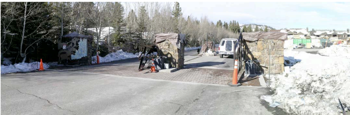
Gate from Ranch Road facing North
